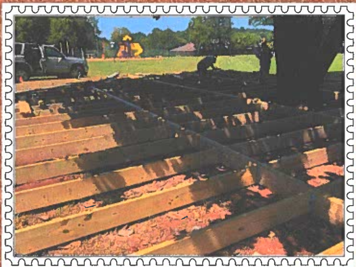
Framework in place.
